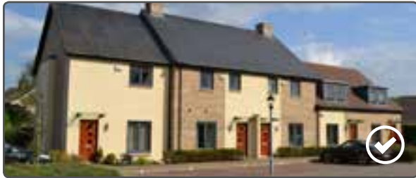
The repetitive nature of this chimney design contributes to the success of this design
