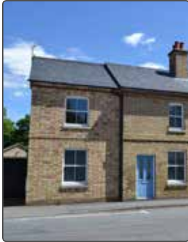
This extension broadly follows the original building line but with a very small set back - Brampton
