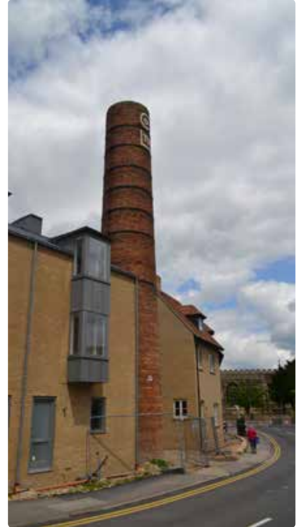
Retention of chimney in new development
