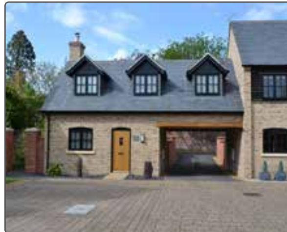
This development in Brampton uses a discreet archway to access some car court parking to the rear, retaining the continuous arrangement of the building form
