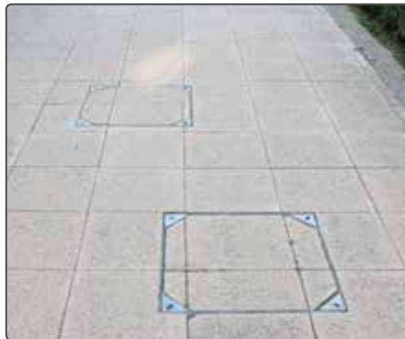
Discreet drain cover within paving, Walden Walk, Huntingdon
