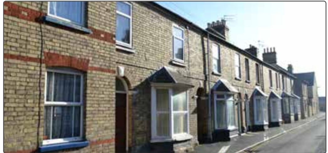
This repetitive window pattern of bay windows adds character to the street - Huntingdon
