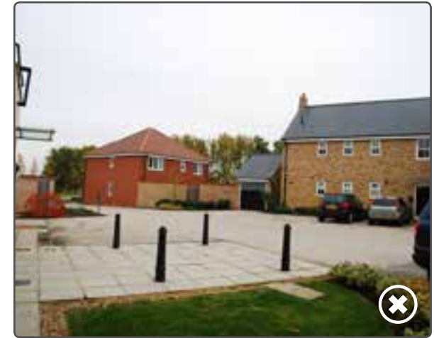
This is a poorly designed car court with ill defined fronts and backs
