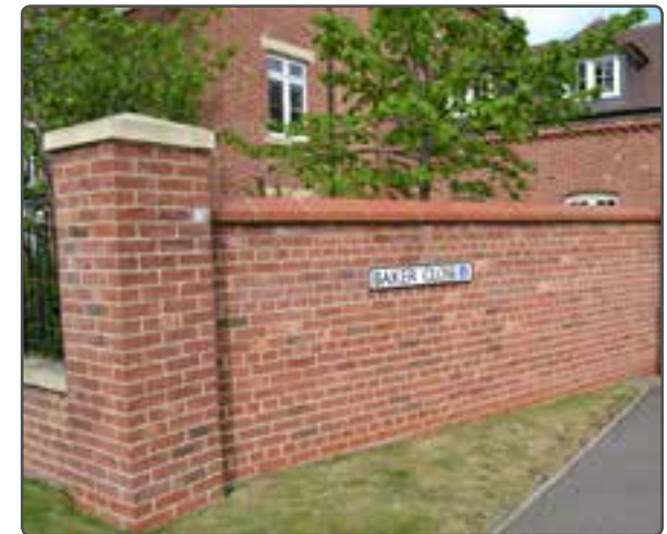
This wall is well detailed and finished - Brampton
