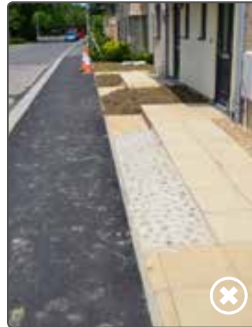
Problems with getting the building threshold sorted out at the end have resulted in a poor solution here
