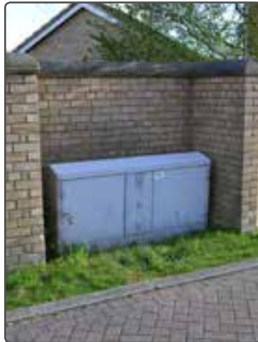
Cabinet hidden behind a reveal in the wall
