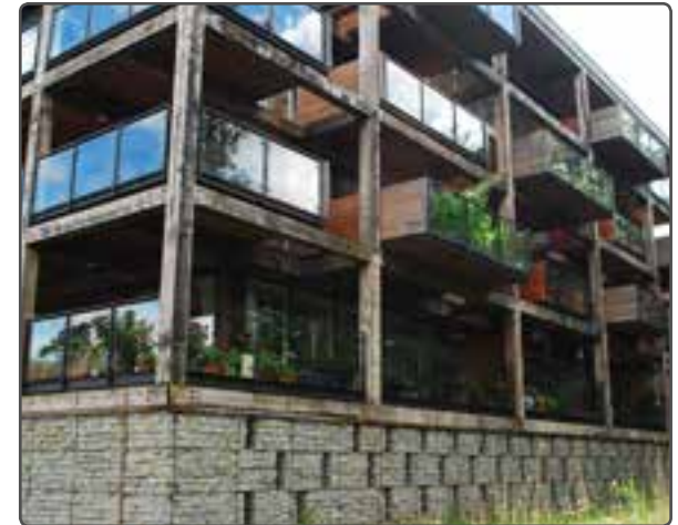
This building uses semi basement parking behind gabions that are designed to let natural light in
