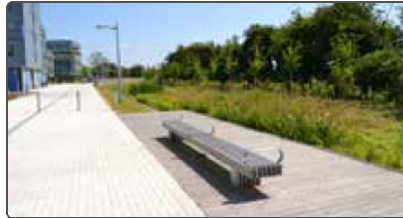
Drainage channel following pedestrian route
