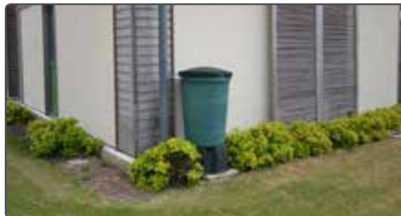
Water butt - rainwater harvesting
