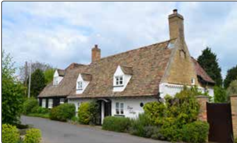
These dormer windows sit lightly on the roof of this cottage - Holywell
