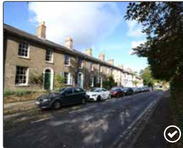
Attractive relationship between buildings and street.
