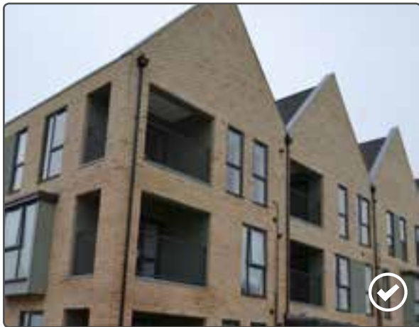
Substantial internal balconies
