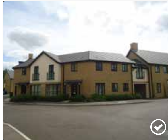
Successful building frontage - Little Paxton
