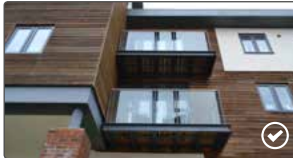
Deep external balconies
