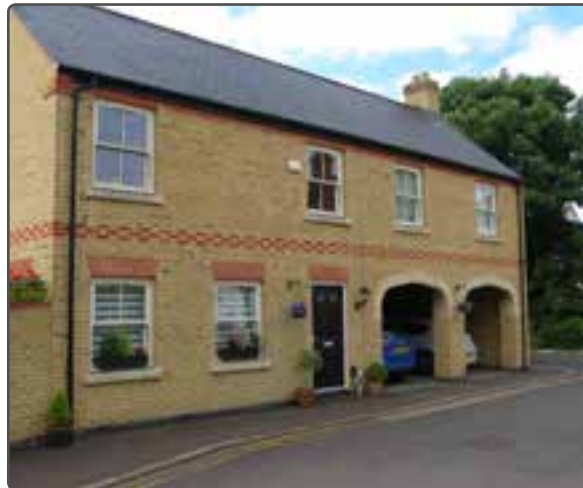
Slate roof at Temple Close, Huntingdon
