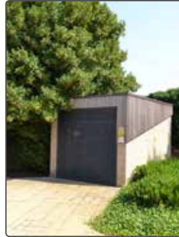
Substation clad in contemporary design
