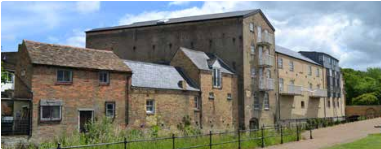
Reuse of former mill building and reinstatement of 3 and 4 storey development adjacent to Hen Brook
