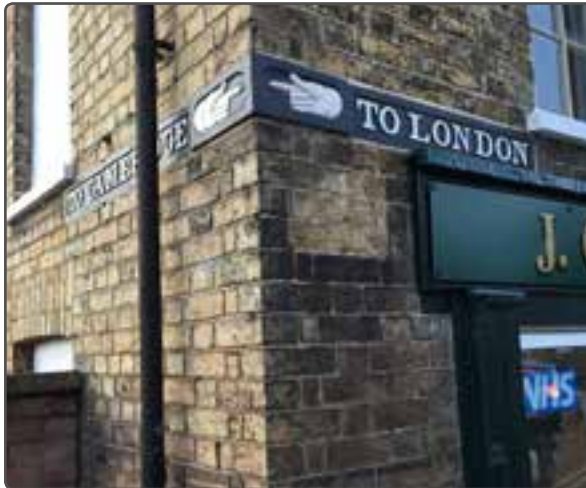
Direction sign attached to building
