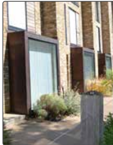
This corten steel window has a deep projection that adds interest to the building
