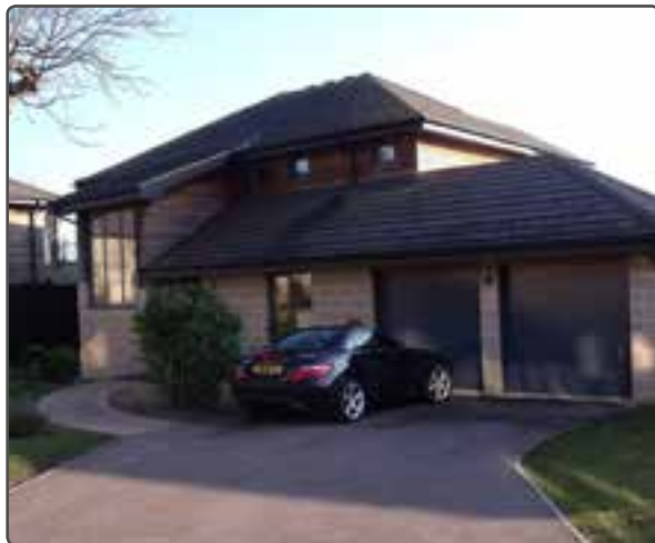
The impact of the double garage is minimised by the overall design of the building
