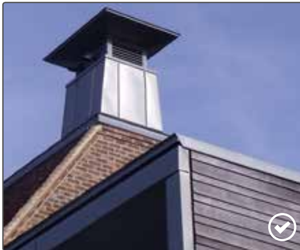
A good example of standing seam used on this ventilation chimney, Cambridge
