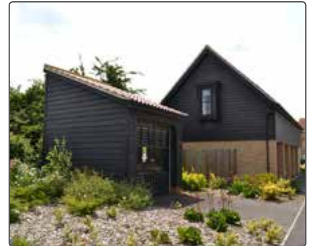
Substation design reflecting adjacent building
