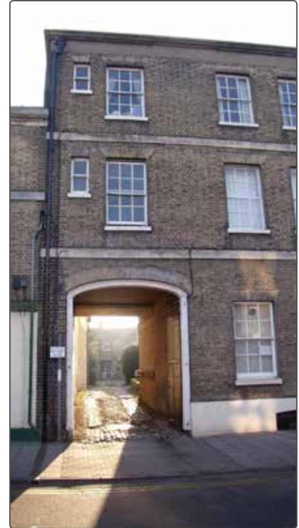
Tall buildings can help to create a sense of place - St Ives
