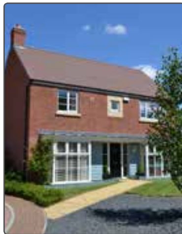
Large ground floor windows enliven this house
