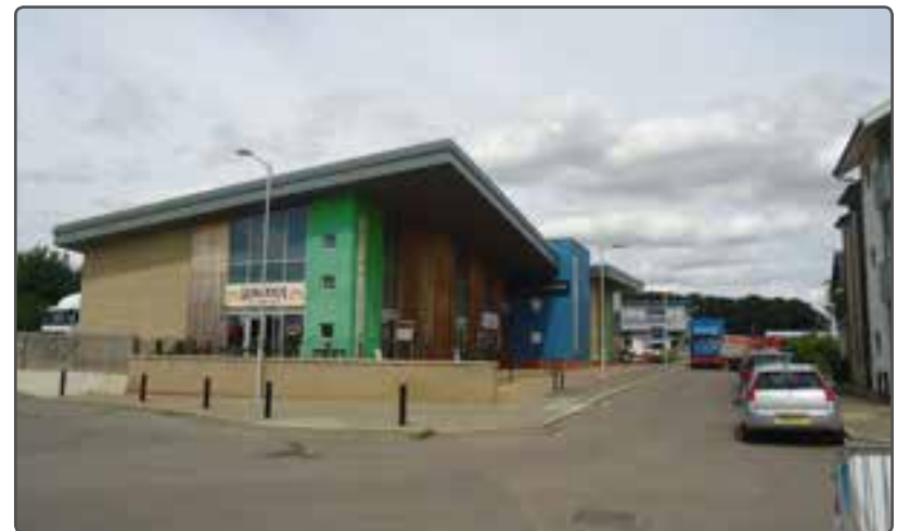
Dual aspect frontage at the mixed commercial development - Loves Farm, St Neots
