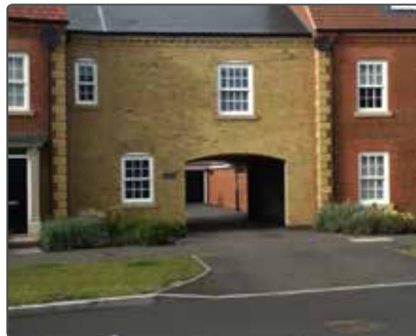
This archway provides access to a rear car court while preserving the continuous building line
