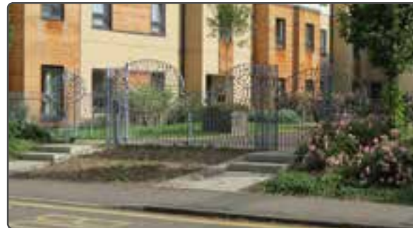
Railings and gates fronting Brookside, Huntingdon
