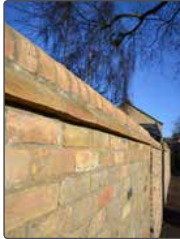
Well detailed brick wall
