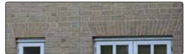
Detail of brick arches
