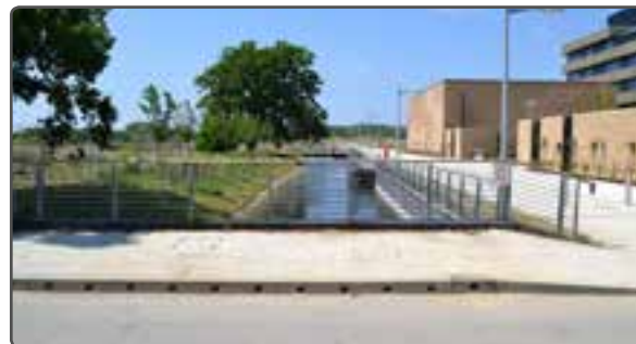
The stream is canalised at this point
