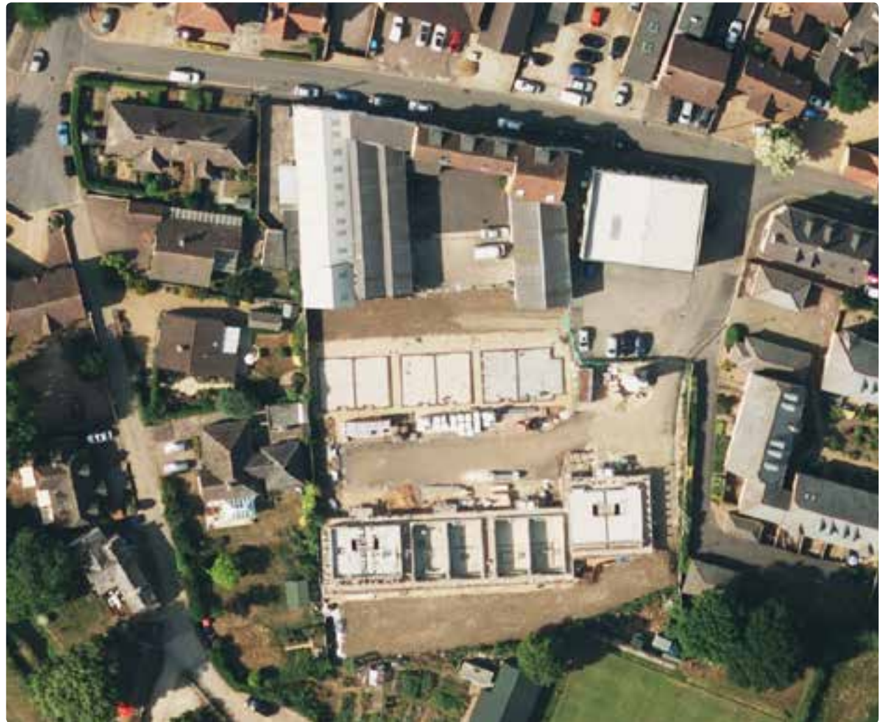
Small group under construction in St Ives
